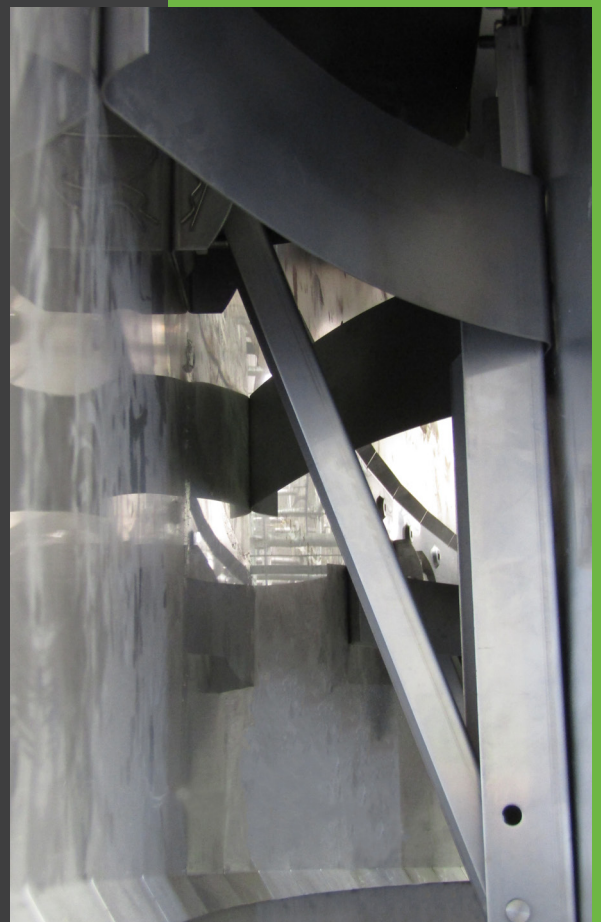
Inner Shoe Primary Mechanical Shoe Seal
